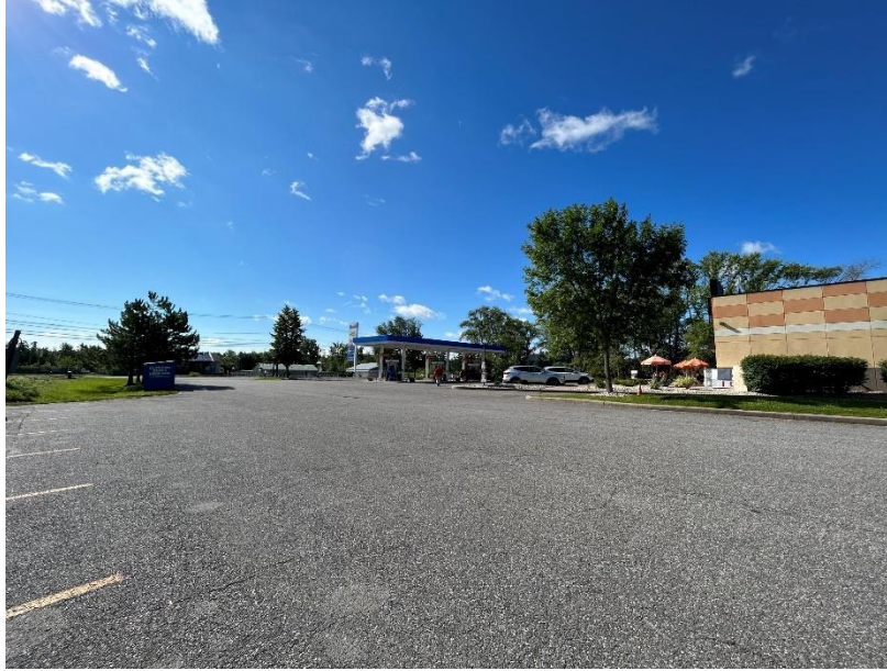
Figure 4.4. The Mountain Mart Parking Lot.
