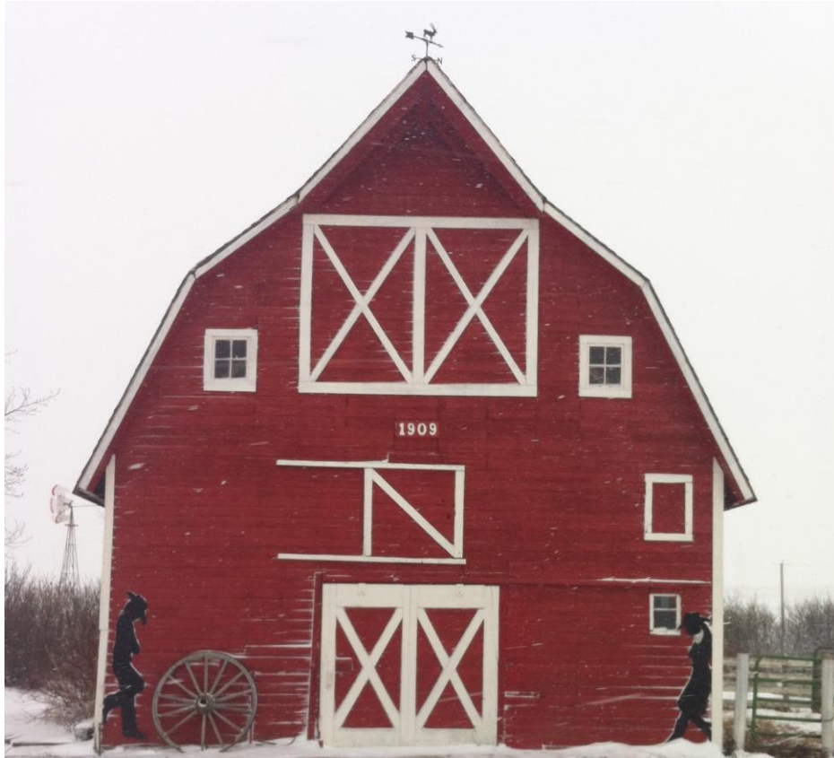
Figure 4.8. Foundations: Etzikom, AB, January 3, 2014
