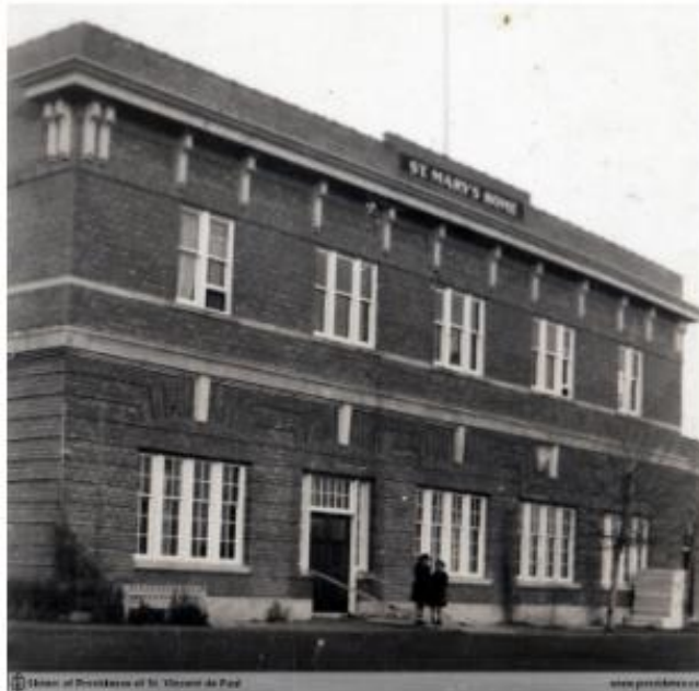
St. Mary's Home after the renovations, ca. 1941 (SPSVPA 014-205.1.2-10)
