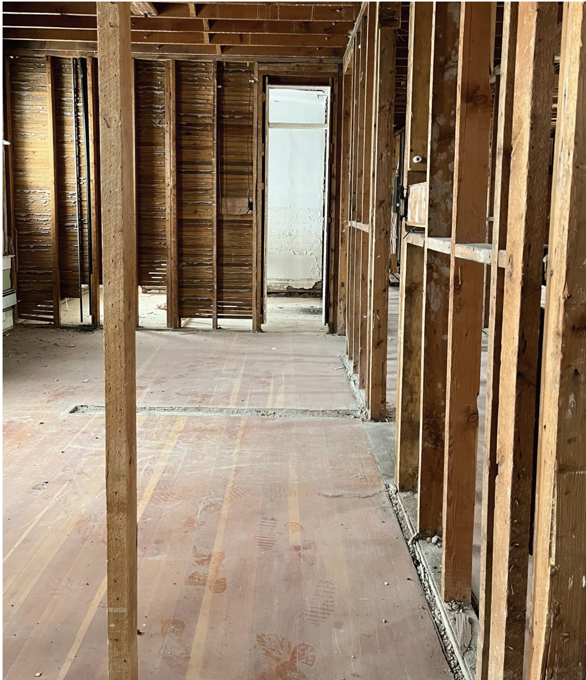
Figure 4: Third Floor Renovations, 17 December 2022
