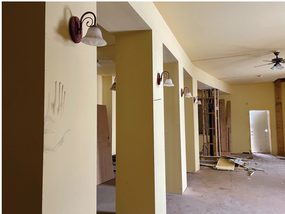
Figure 2: American Hotel Main Floor, 17 December 2022
