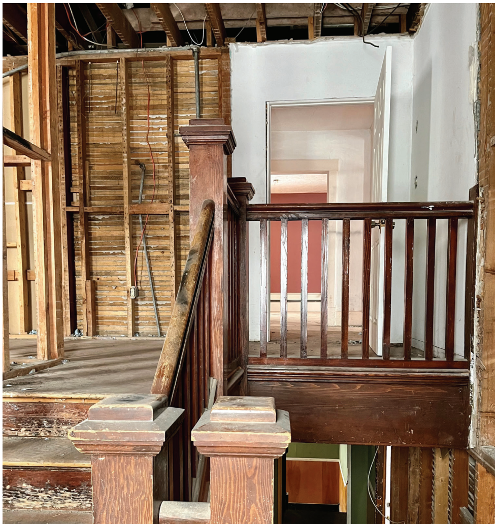
Figure 5: Third Floor Staircase, 17 December 2022
