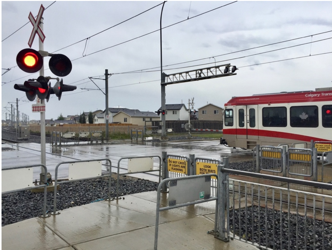
Figure 4.12: Level C-Train crossing in Martindale
