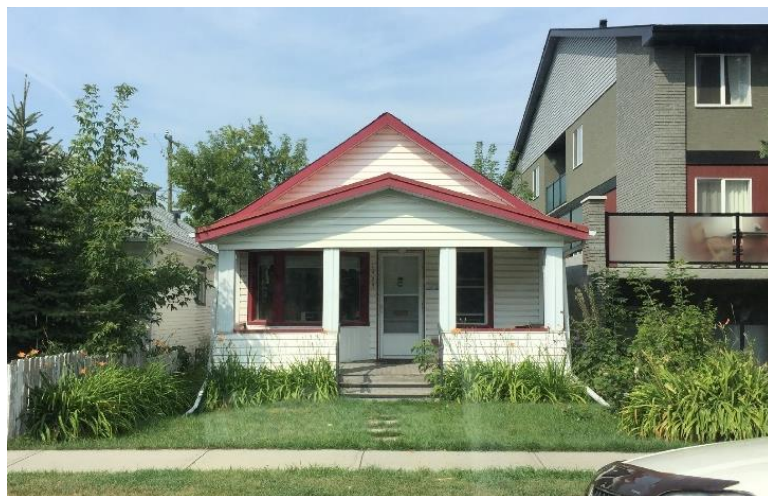
Figure 4.28: Older Single-family House.
