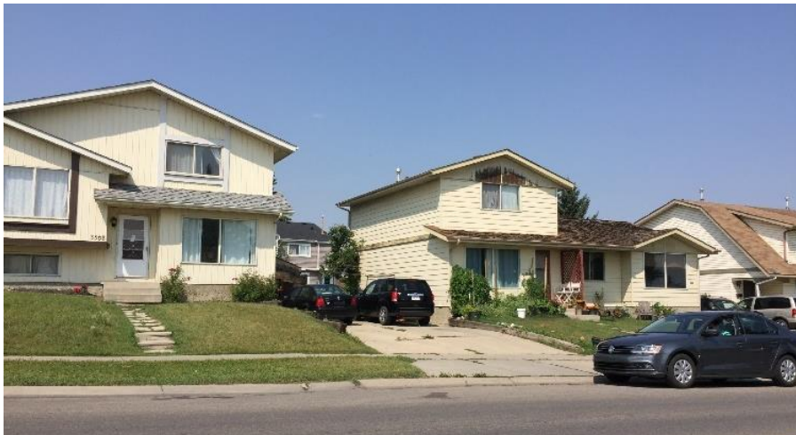
Figure 4.29: House Needing Small Repairs Such as Painting.
