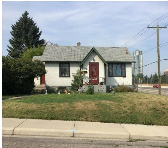
Figure 4.24: Old Single-family House with Stucco Facade.
