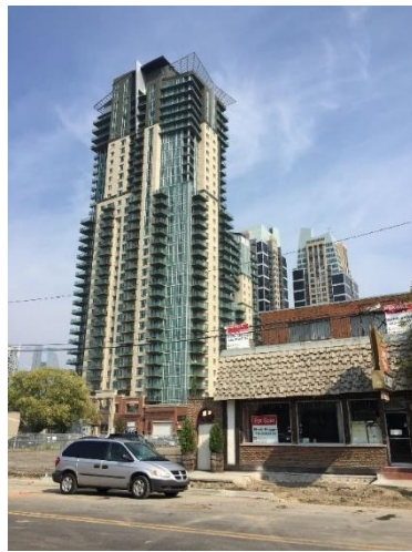
Figure 4.17: Contrast between New High Rise Residential Towers and Older Dwelling
