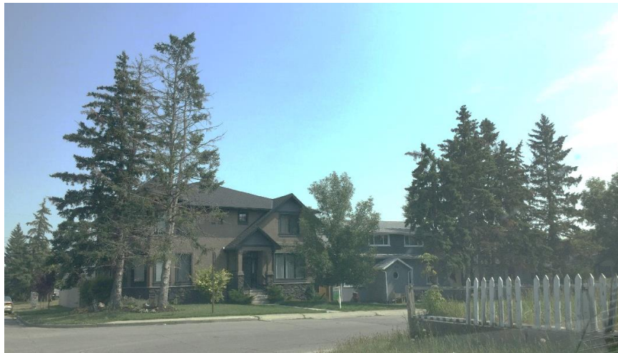
Figure 4.39:Single family House.
