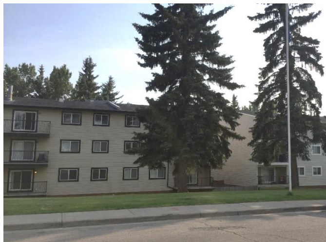
Figure 4.53: Low Rise Apartment Buildings.
