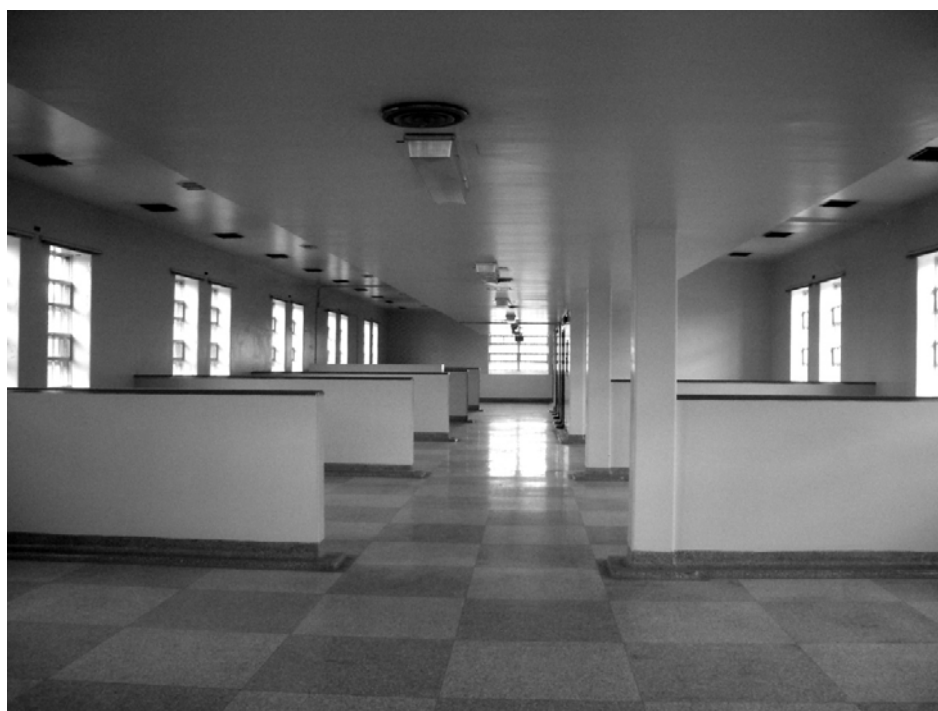
Figure 4. A typical ward, Michener Center.
