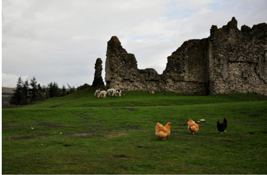
Figure 20: Bewcastle Castle, looking east. Photograph by the author.
