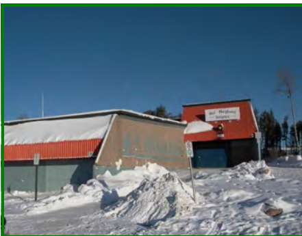
The Uniplex (Evacuation Centre)
