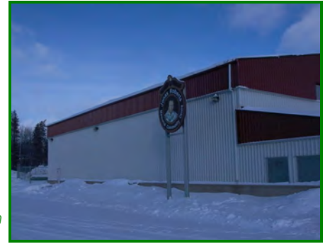
Jonas Roberts Memorial Community Centre Photo Courtesy of J. Kulig
